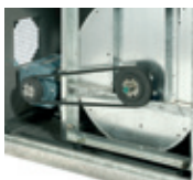
Motor outside the airflow path
