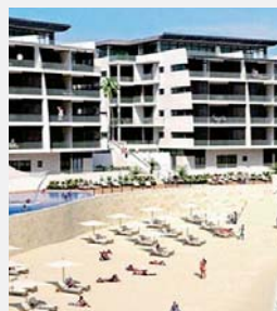
Location: Kenya (Mombasa) Project: English Point Marina
