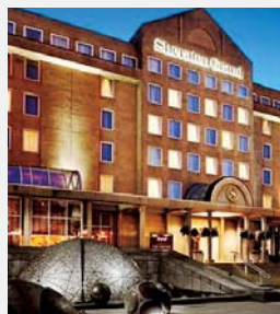
Location: UK (Edinburgh) Project: Sheraton Hotel
