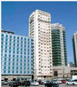
Location: Qatar Project: Office Building
