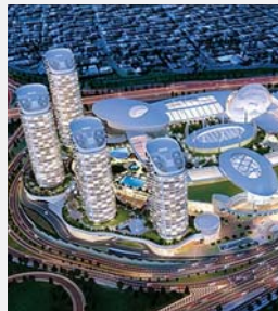
Location: Turkey (Istanbul) Project: Mall of Istanbul
