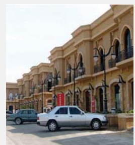
Location: Saudi Arabia Project: Medical Clinic
